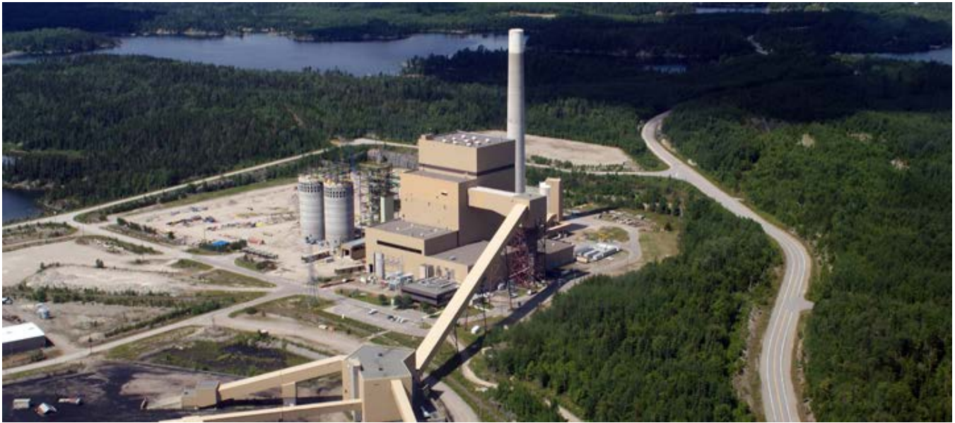
OPG's Atikokan 100% White Pellet Fueled Power Station
